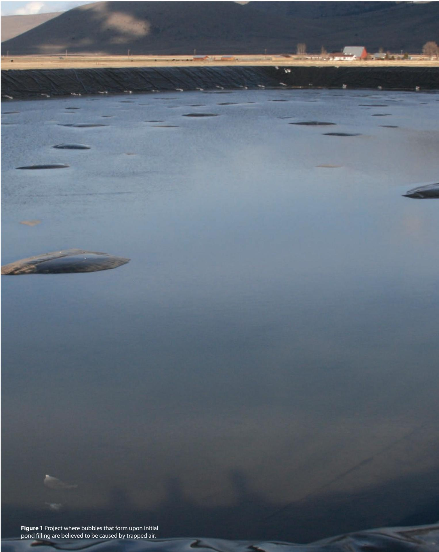
**Figure 1** Project where bubbles that form upon initial pond filling are believed to be caused by trapped air.
