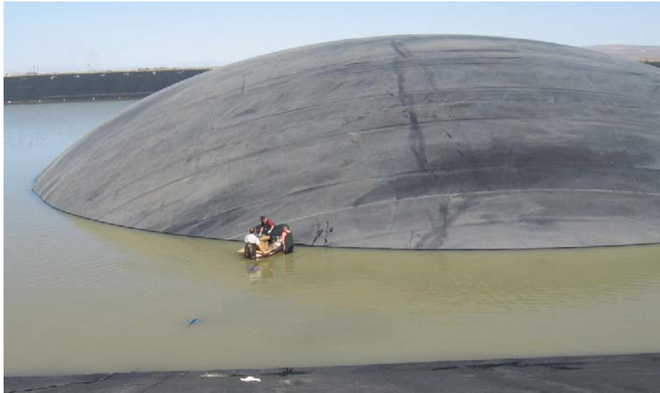
Figure 1: Example of large geomembrane gas bubble (note people in photo for scale).
