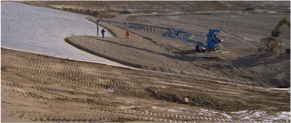
Figure 1. Placing gravel onto PVC with telebelt on 4:1 slope.
