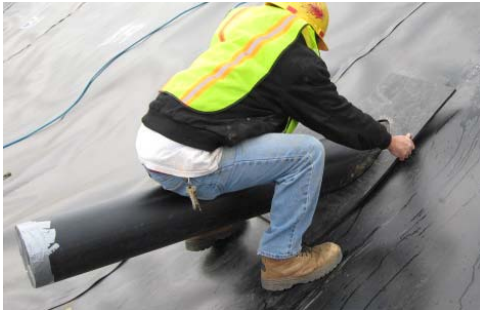
(a) Fitting plate-skirt.
