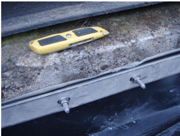
(a) Thick fuel-resistant moldable sealant used to provide leak-resistant seal against rough concrete.
