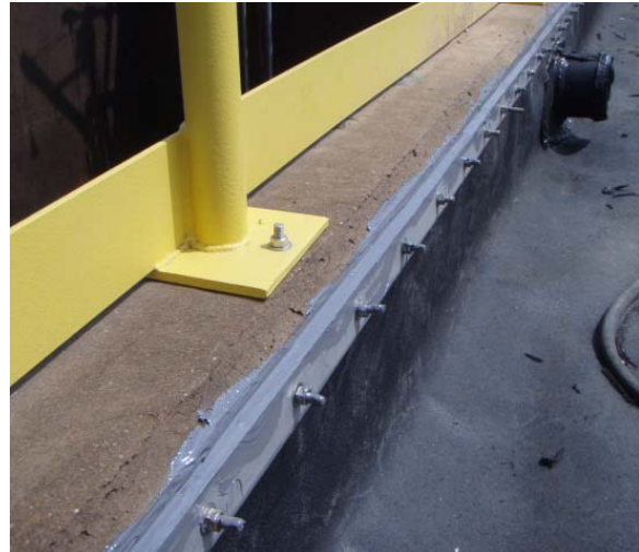
(b) Polysulfide coating over top edge of batten.
