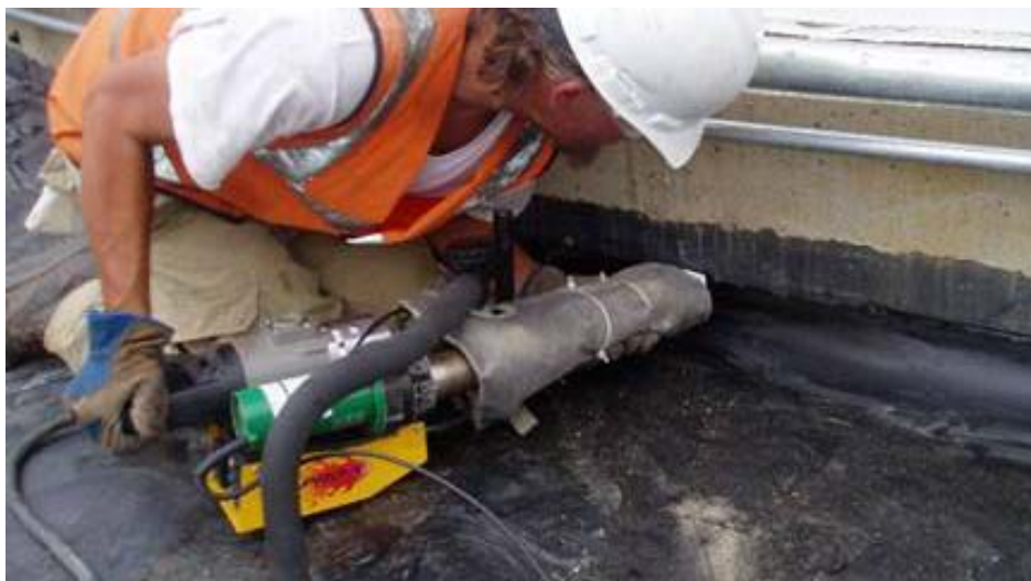
Figure 16. Welding geomembrane to embedment strip with preheater on extrusion gun.
