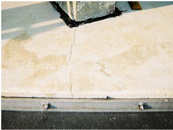
(c) Hairline crack in concrete will defeat batten when submerged.
