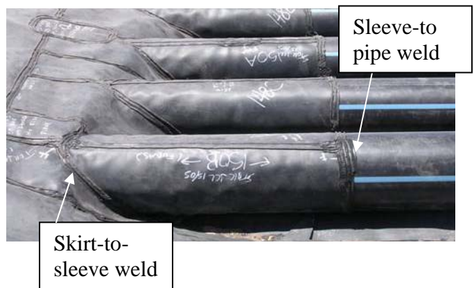
(b) Boot sleeve welded to pipe. This is commonly preferred by many installers for leak resistance.
