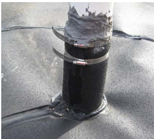
(a) Gasketed and banded boot with polysulfide coating on the end of the boot.
