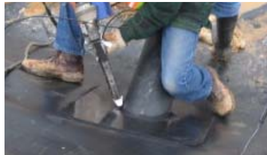
(d) Welding the pipe to the plate. Ideally another welded boot will be installed over this.
