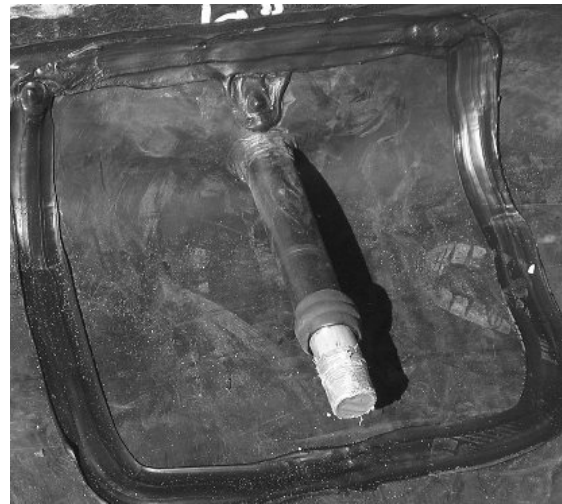
(b) Installed penetration.
