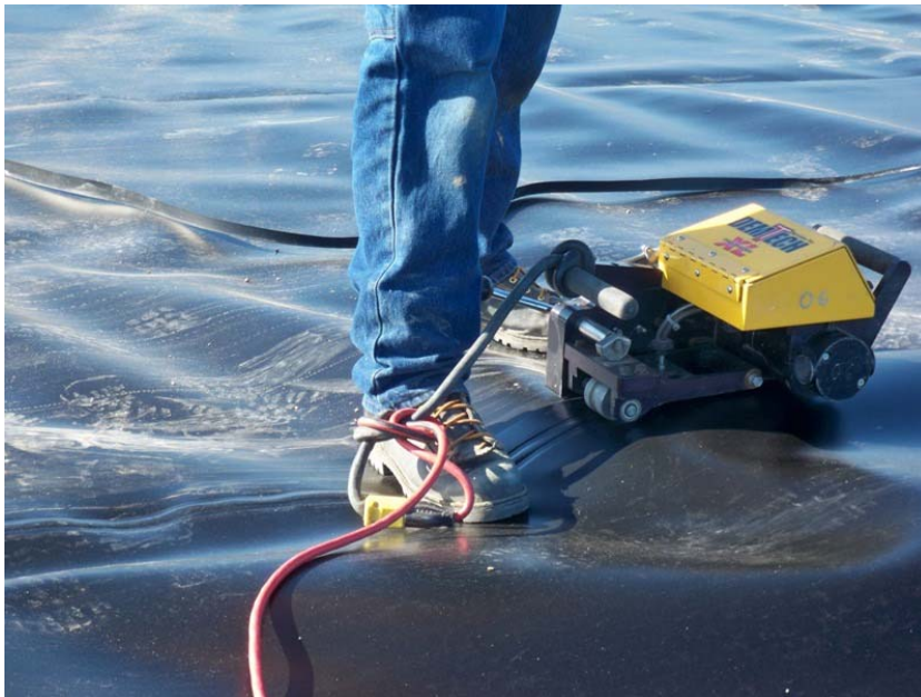
Stepping on the weld just behind the machine, while weld is still hot, to preserve alignment and work with wrinkles
