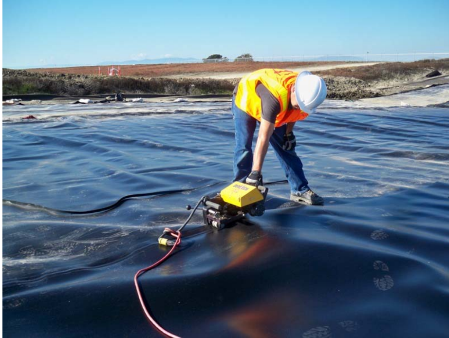
Re-aligning machine during welding
