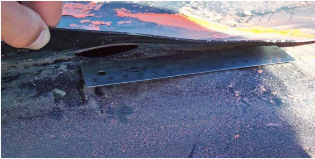
Tear under the flat that would never have been found without water lance survey.
