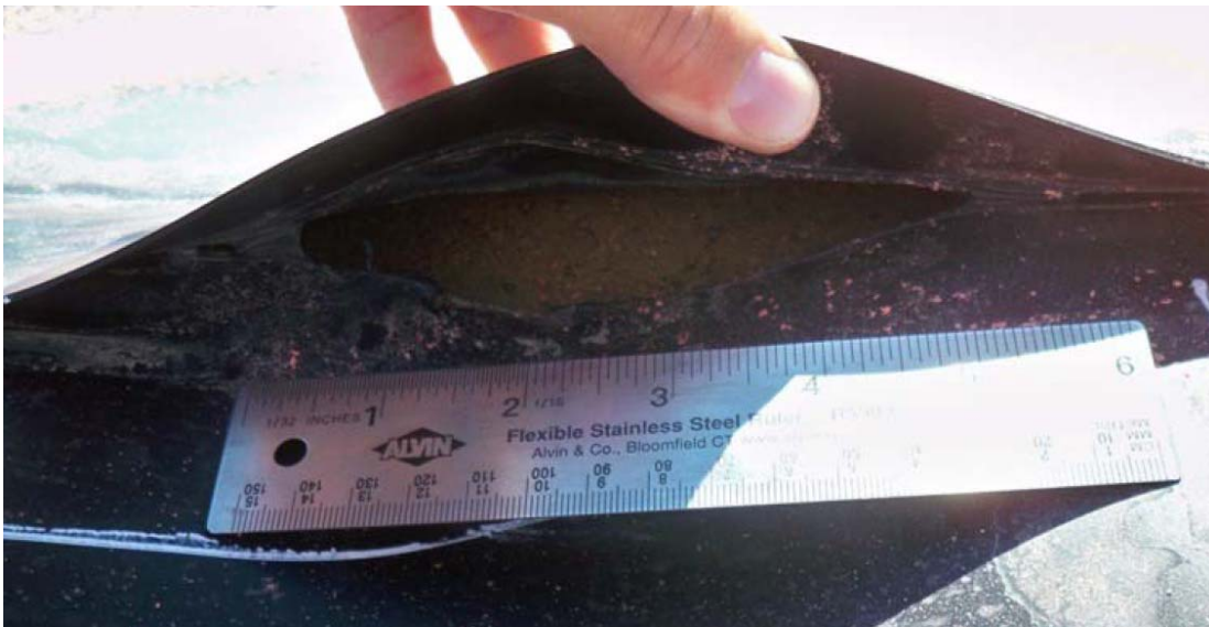
Dramatic example of rip under the flap.
