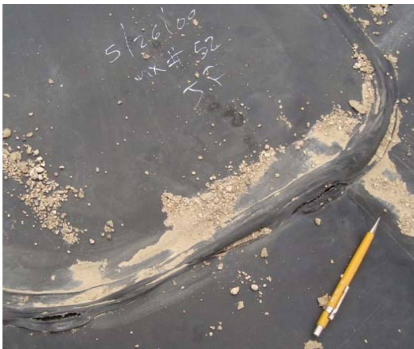
Same story as above – two separate tears in lower sheet. Note QC sign-off on the patch.
